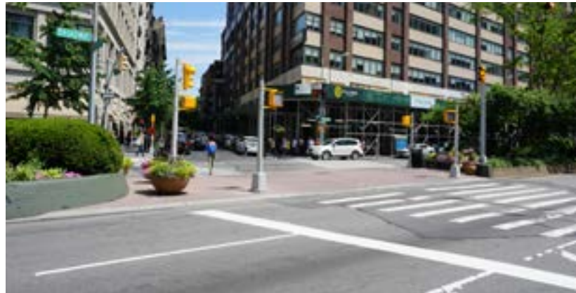
Bottom: Mountable median with brick paving
